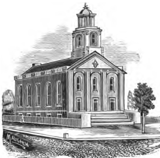
PRESENT FIRST CHURCH, BEFORE ALTERATION.
